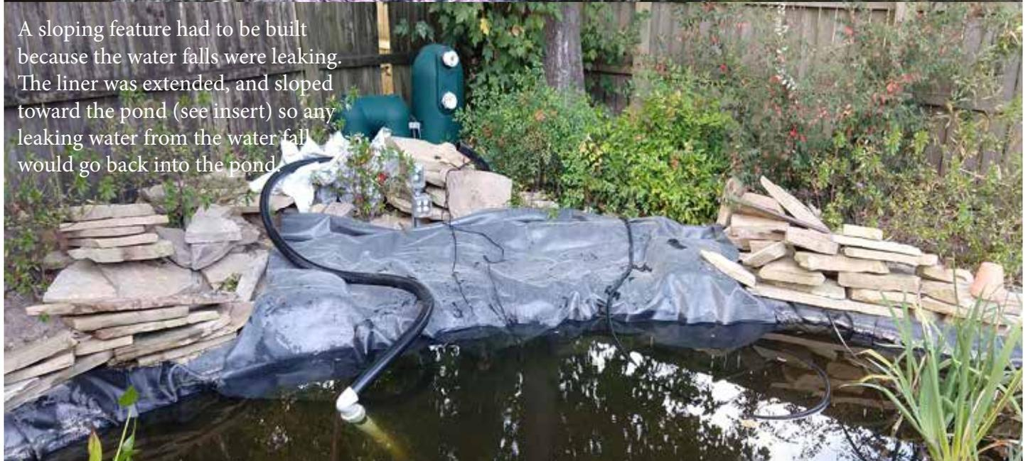
A sloping feature had to be built because the water falls were leaking. The liner was extended, and sloped toward the pond (see insert) so any leaking water from the water fall would go back into the pond.
