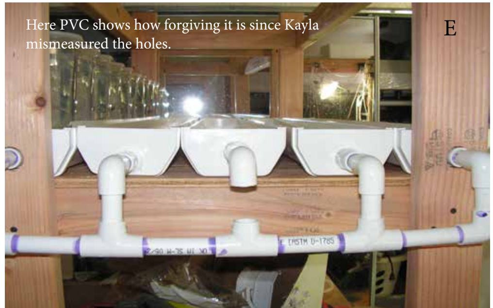
First shelf drain installed. That barbed outlet was later changed for a 3/4 gravity fed pipe.
