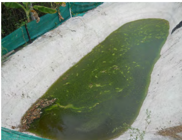
Waste water containment pond.
