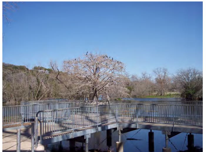
The pier looking out to Pelican Island.
